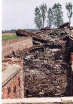
All gas chambers at Birkenau were destroyed by the Nazis. The picture above shows the ruins of one of the five crematoria.
