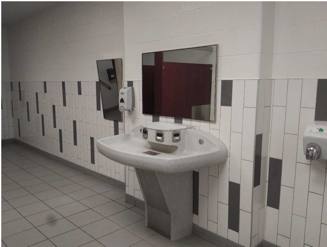
Figure 6. Typical student washroom wall tiles.
