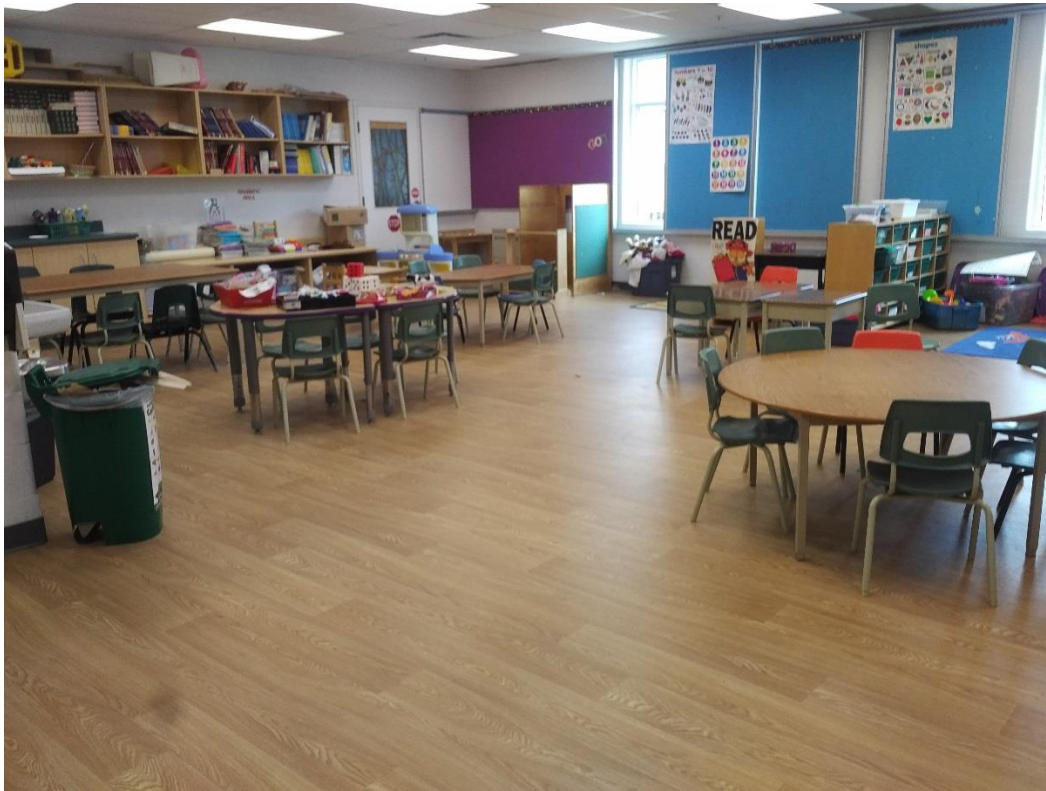
Figure 1. Typical Kindergarten Flooring Replacement
