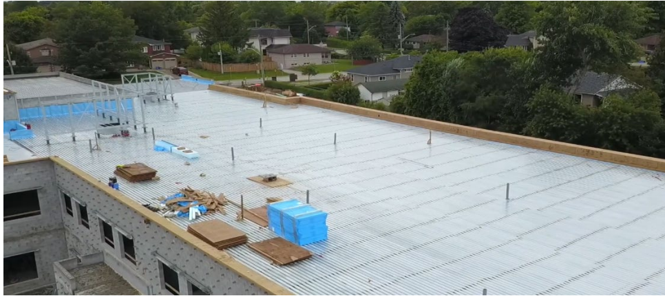
St. Nicholas CES Roof
