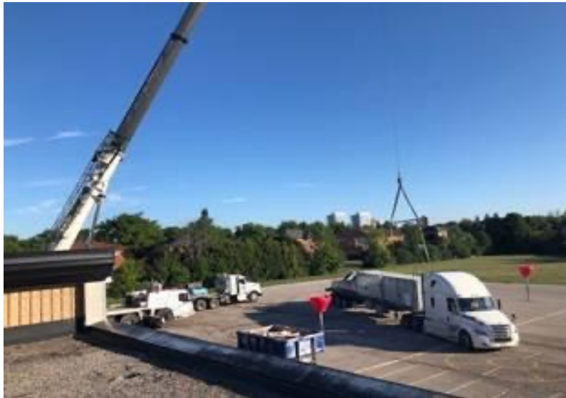
Rooftop Unit Installation at Thomas Merton Centre (Oakville)
