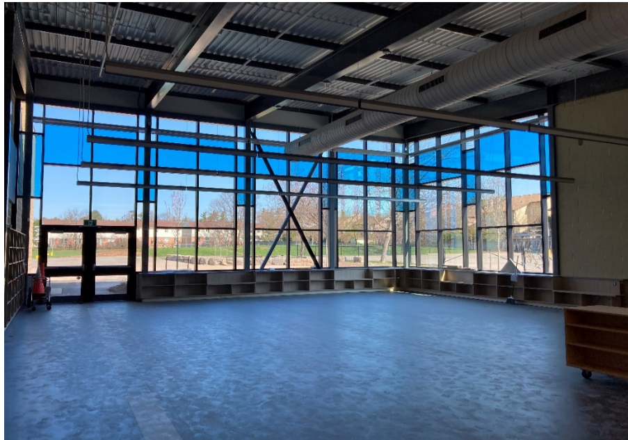
St. Michael CES Learning Commons Addition
