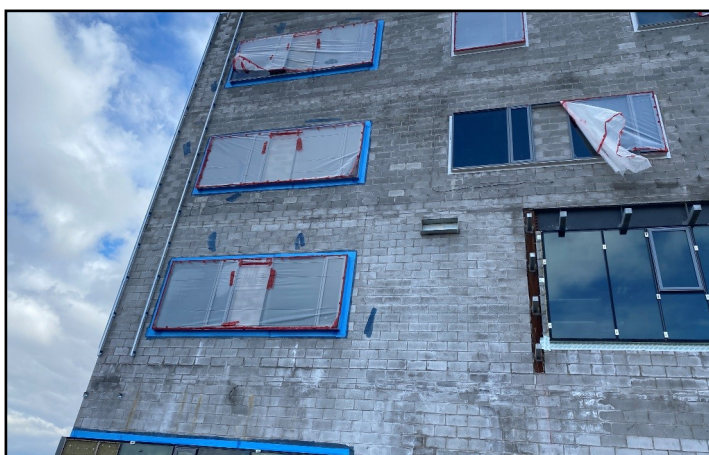
Air-vapour barrier being applied around the windows.
