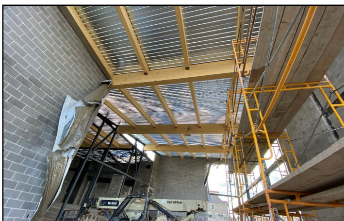
Glulam beams and metal decking have been completed.
