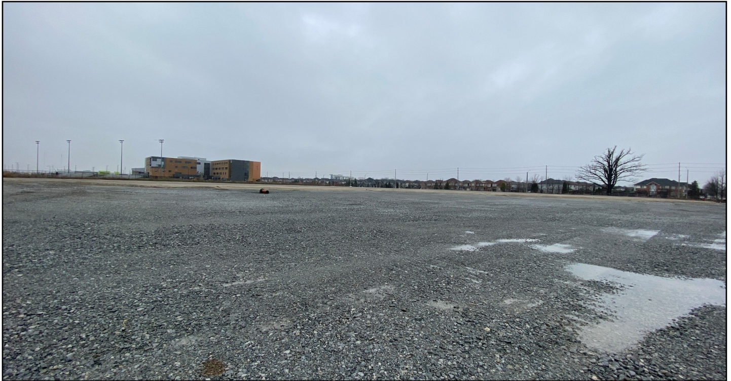
Building site pad.
