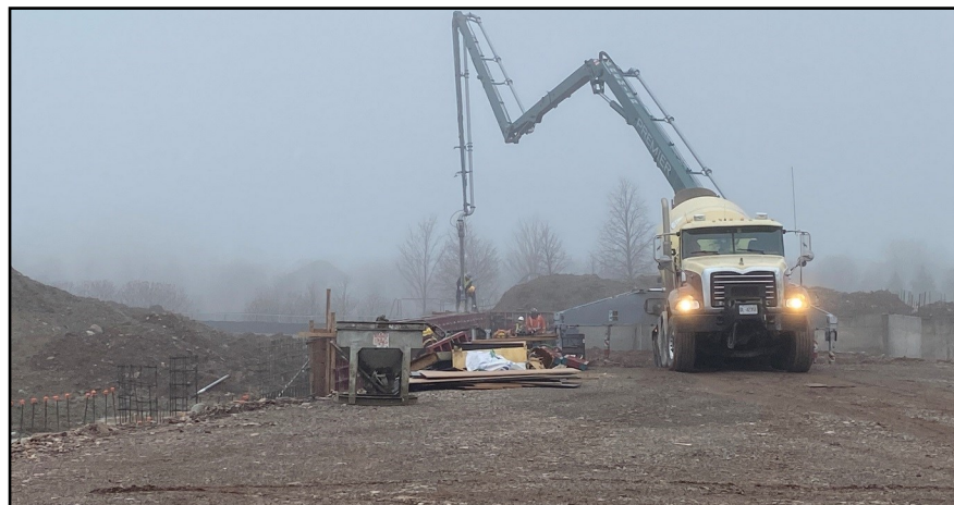
Foundation walls being poured.
