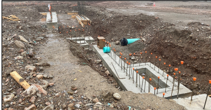
Footing installation underway.
